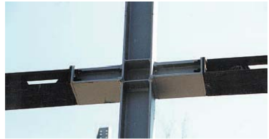
Figure 8: Gooseneck column used in Girder-Slab construction
